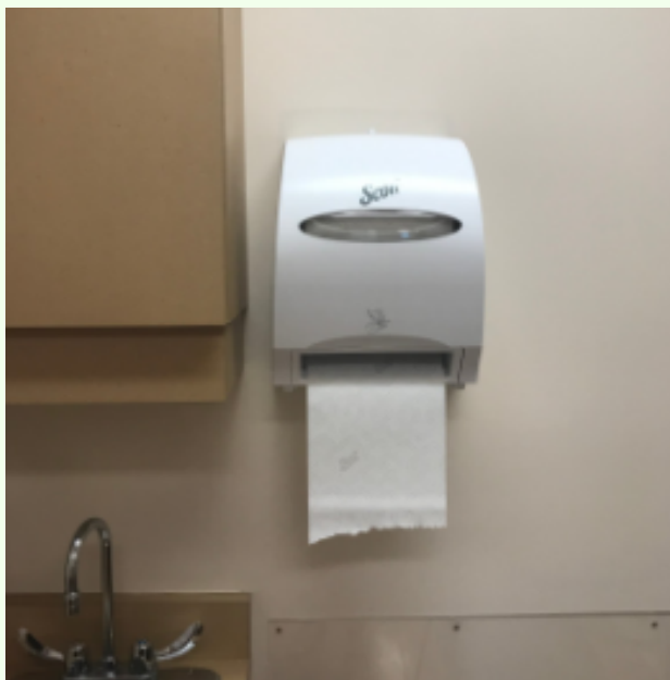
Our new dispenser in an examination room.
