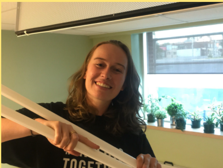
Rebecca Gillet Installing LED Lights
